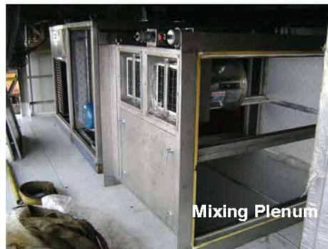
Air Cooled Packaged Unit
